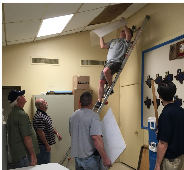
Brothers Jerry McGee, Francis Rotering, Chuck Clark, and Steven Barmore help out from below as Neal Hoelting starts on the last ceiling tile.
